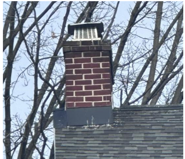
Second masonry chimney on roof
