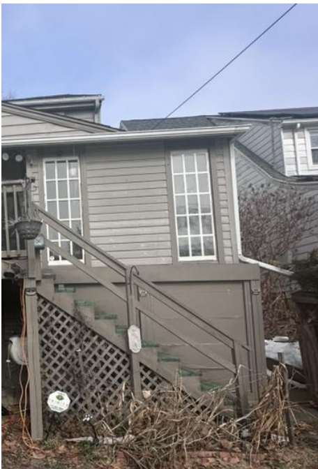
Wooden stairs consisting of tread, risers, and a balustrade.
