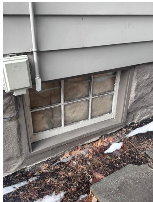
Basement level window opening
