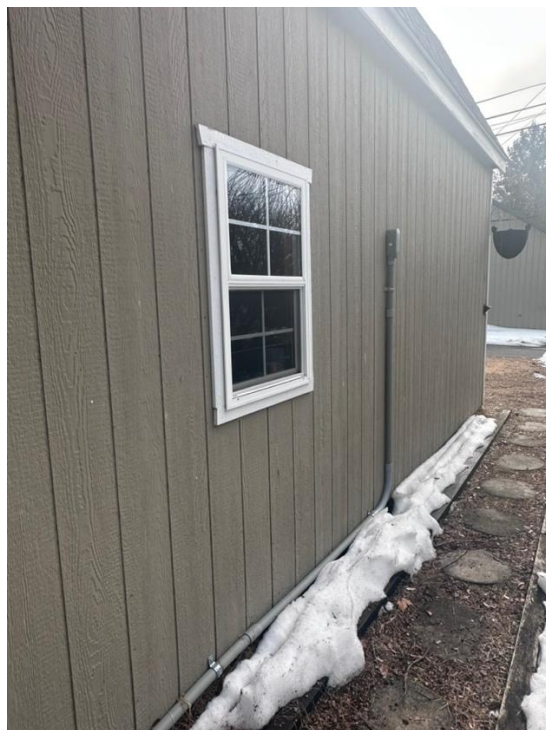
Double-hung window with a multi-pane sash configuration
