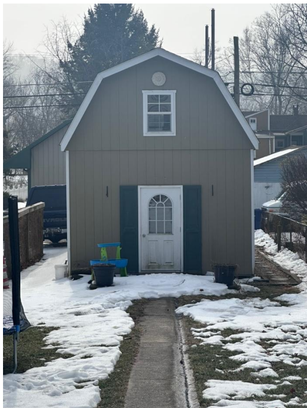
Façade of rear building
