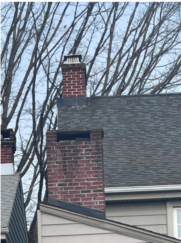
Photo to show both masonry chimneys
