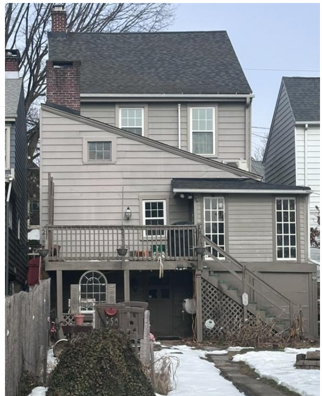
Rear view of the house
