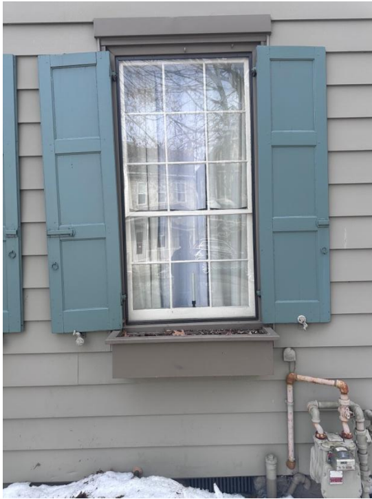
First story window with solid shutters
