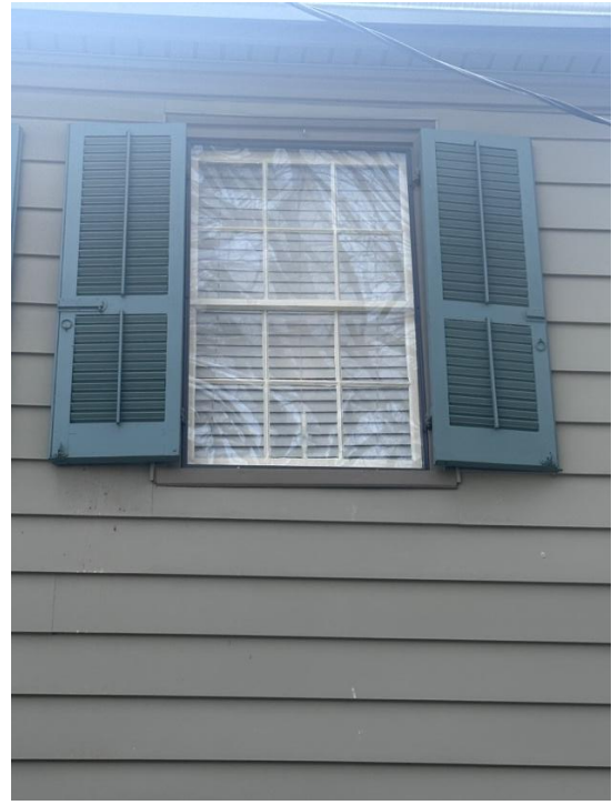
Second story window with louvered shutters
