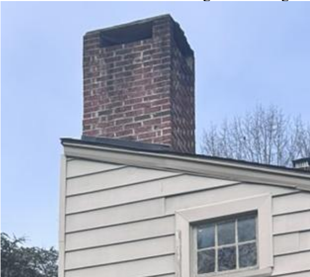
Masonry chimney on rear of the house
