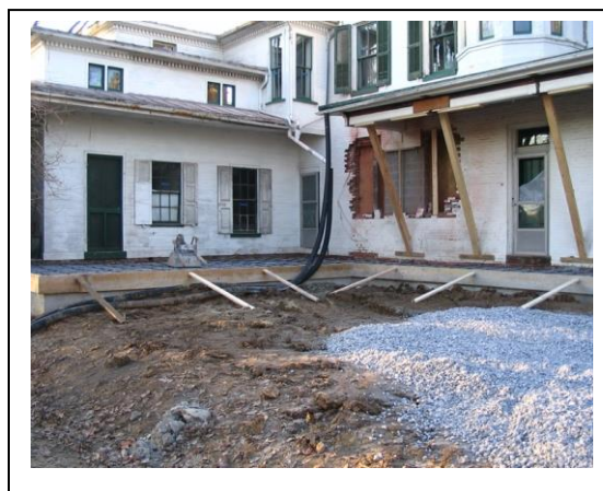
Extending the porch on the backside of the Barr Spangler Manse.
