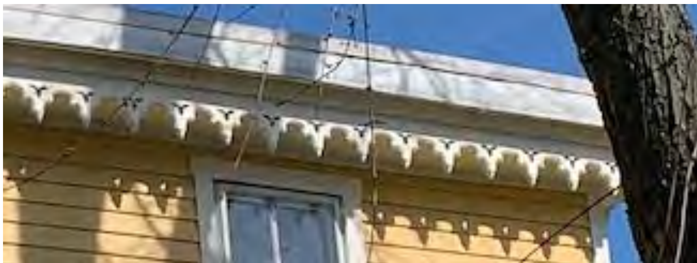
There is dentil work located along the roofline of the whole house.
