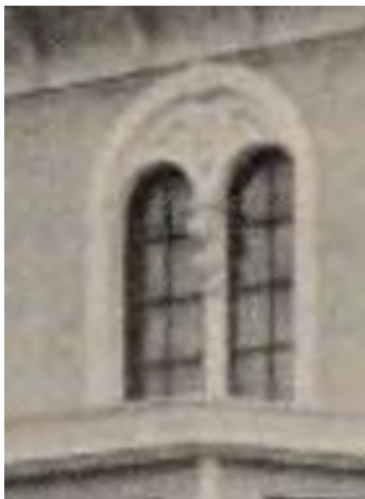
On the old square tower were tall, narrow windows with curved arches. This is consistent with the Italianate architectural style.
