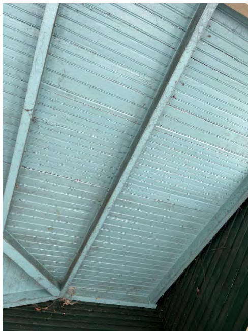
Paneling on the roof of porch in front of the house
