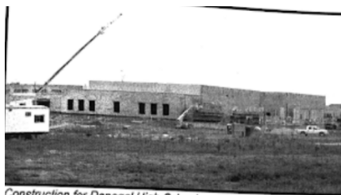
Construction for Donegal High School
