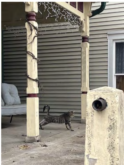
Balusters located in the front of the house, supporting the porch. Balusters are vertical members or posts.
