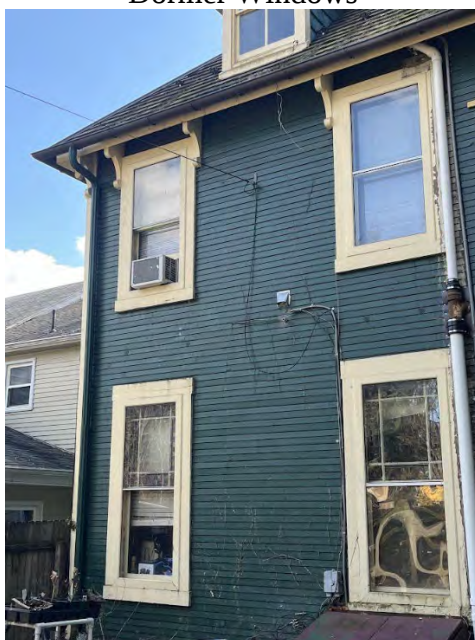
Back side of the house
