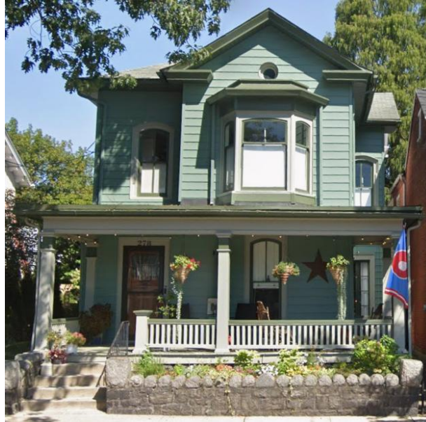
The house features a portico porch supported by tuscan style columns and square balusters forming a balustrade. The roof is hipped.
