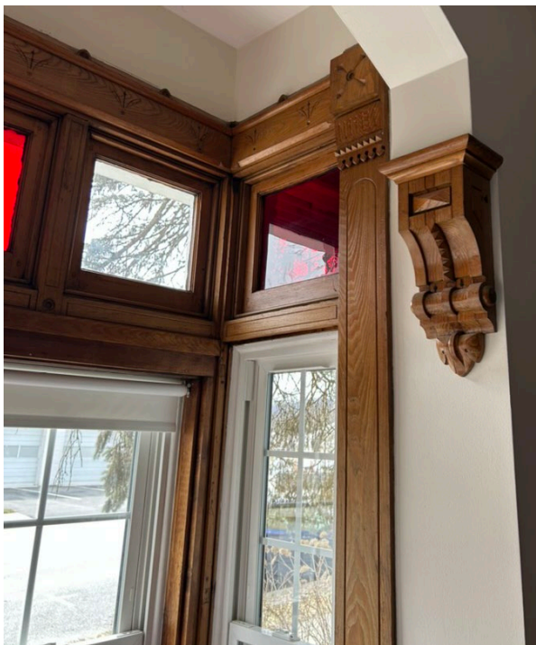
Wood trim along window with lintel above
