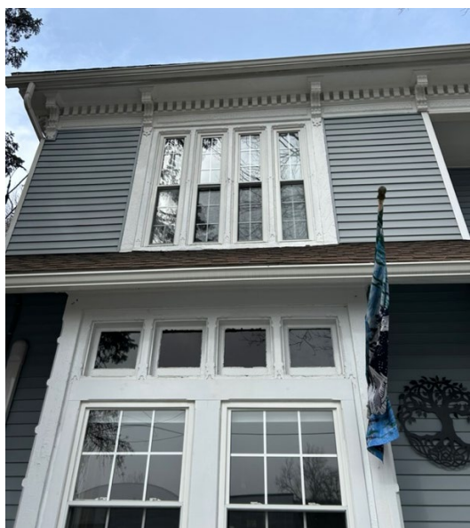
Pent roof + Cornice adjacent to roof
