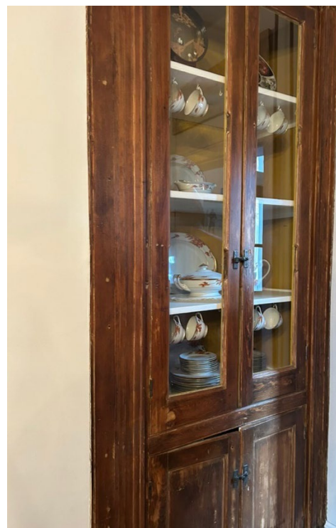
Built in Wooden cabinets
