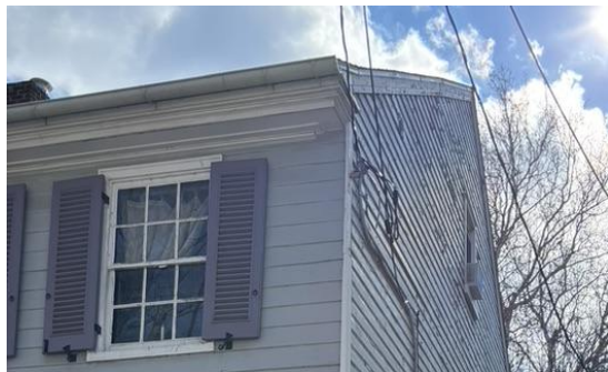
Can see the shape of low pitched side-gable roof.
