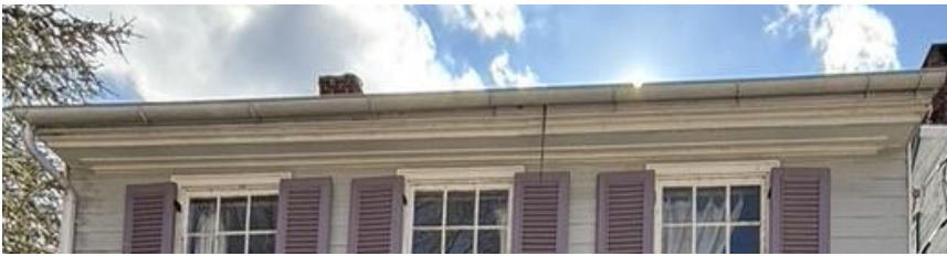
Left: Cornice with molding just below the roof.
