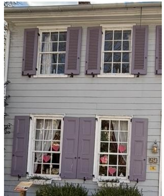
Right: Double hung windows with thin muntins separating panes. Top windows follow 6 panes over 6 panes, bottom windows contain 9 panes over 6 panes
