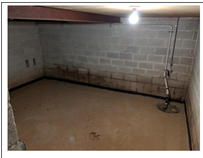
Image of the property's basement bomb shelter, built sometime after 1940. The room was built below the waterline and often filled with water. Photo taken February 11, 2020.
