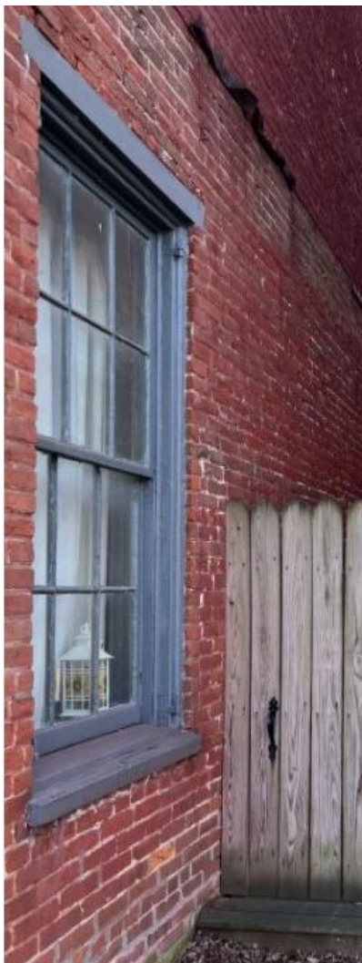
Double hung windows with thin muntin's separating the panes
