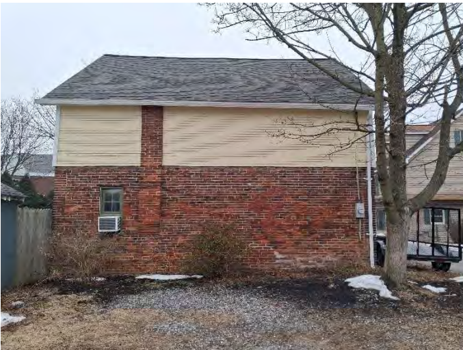
West side of carriage house
