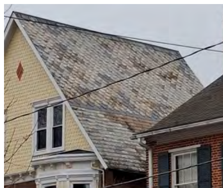
Patterned shingles (west side)
