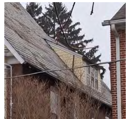
Shed dormer on the west side
