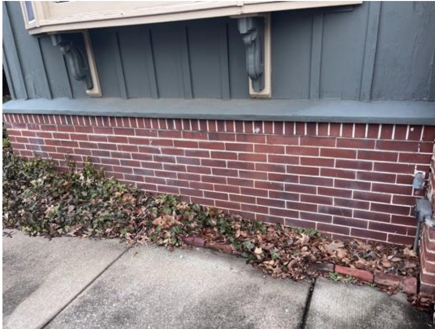
The foundation has masonry brick construction.
