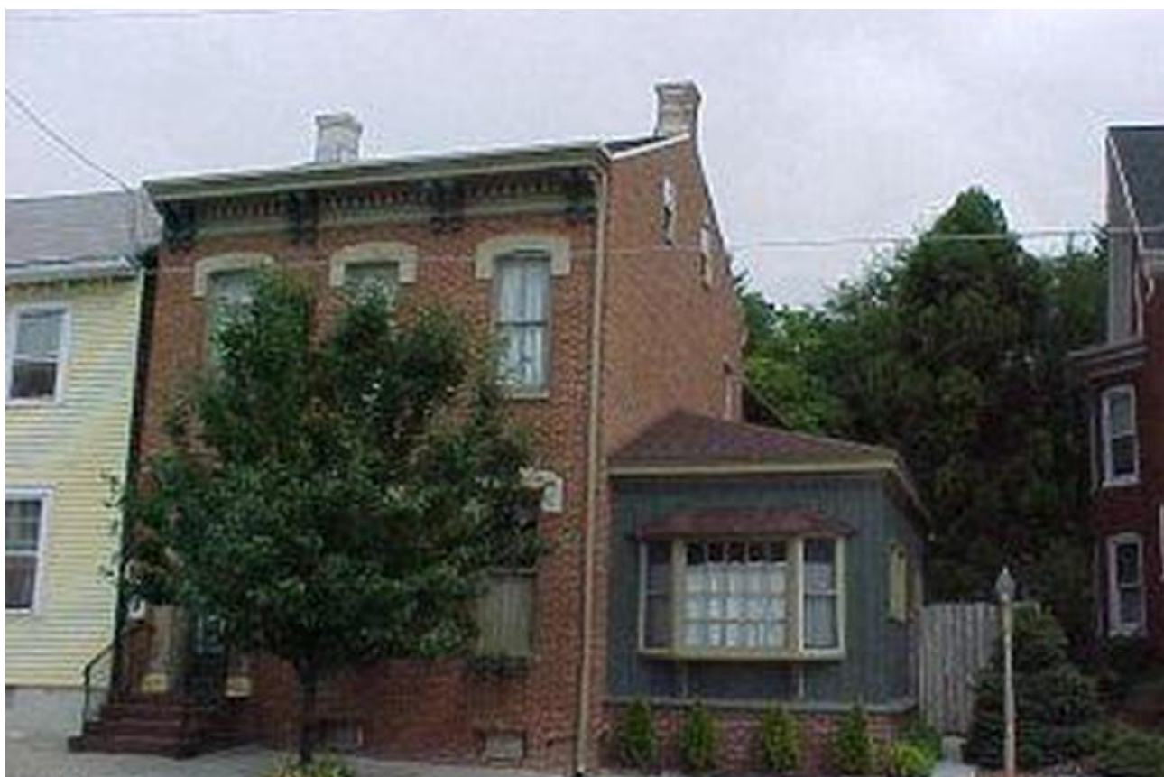
The house had a bay window. The window had 20 panels which were two- one over one.
