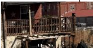
Balustrade on back porch
