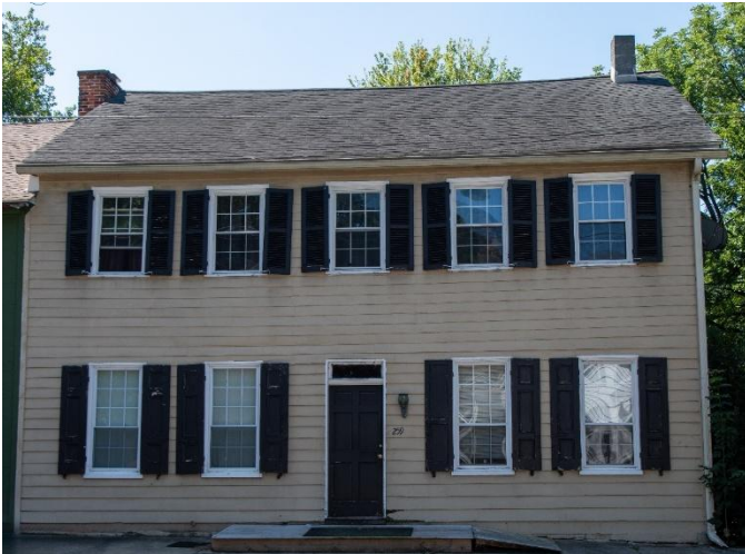
Five Bay Facade
