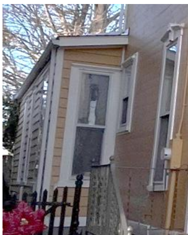
There is a bay window along the left side of the house. The balustrade leading up to another entryway is a twist design.
