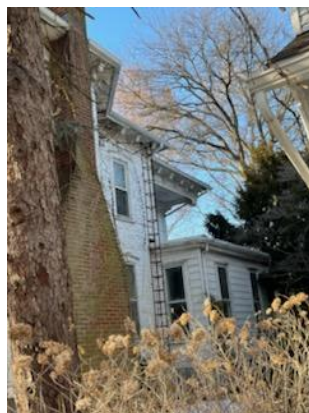
The brick chimney appears to be Flemish bond style. There is another bay window off the back.
