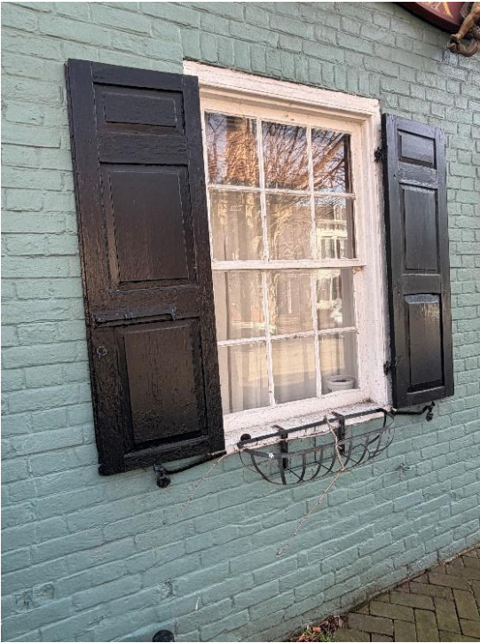
Street level window
