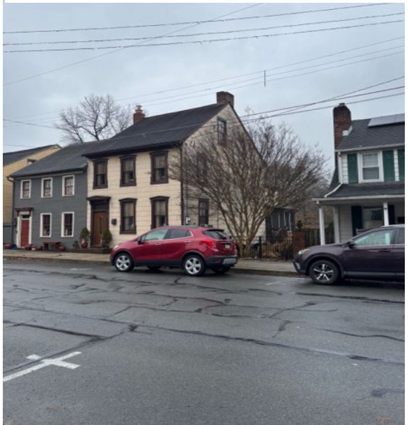
Gable roof, wood frame porch and one-story addition behind
