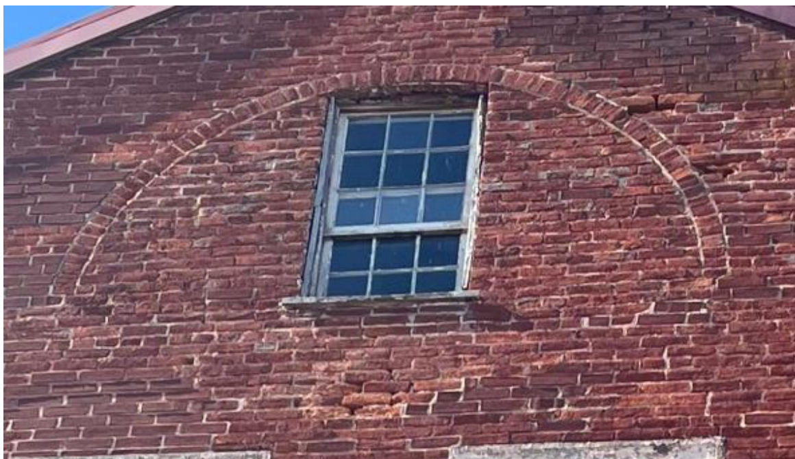
Blind arch above the top window. There used to be a Poladian window in the markings above the window.
