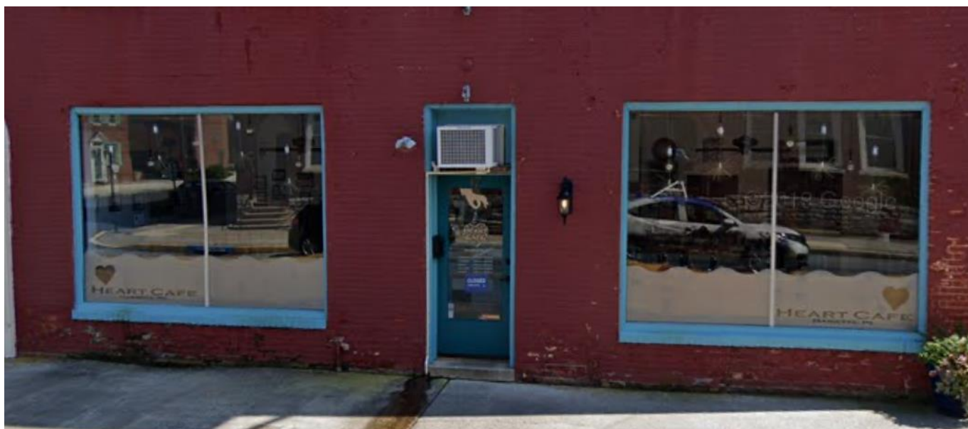
Store front at ground level of the building.
