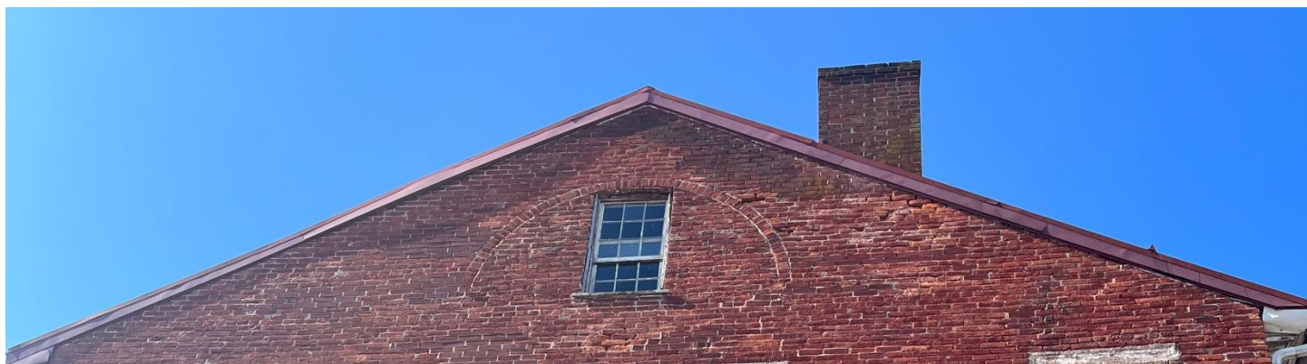
Roof type built is open gable.
