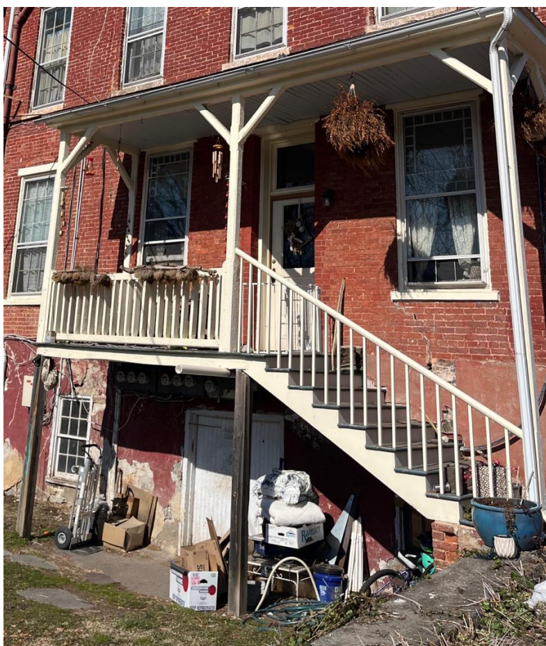
Victorian style porch with balustrade and open string style railings on the stairs.
