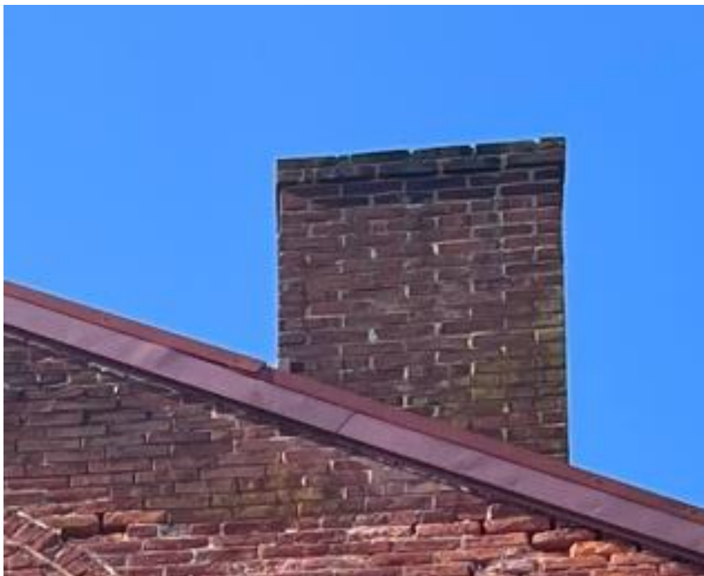
Chimney built using brick
